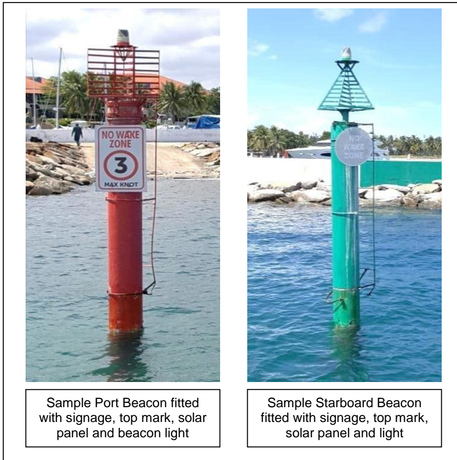
Plate 8: Photographs of port and starboard guide beacons at Sutera Harbour breakwater entrance
