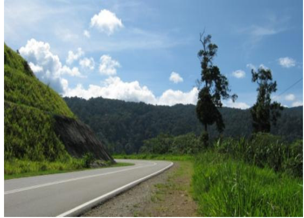
Plate 4.10-9 Access roads Road cutting through Gunung Lumaku Forest Reserve
