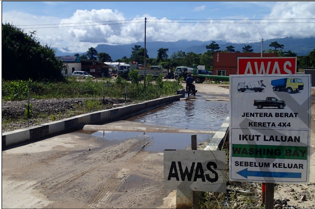
Photo 35 Example of wash bay at the entrance of the construction site.
