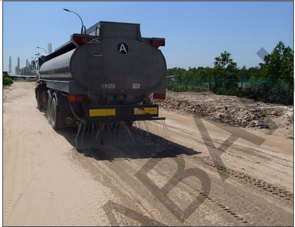
Photo 34 Example of water tanker with sprinkler system to dampen the road access.
