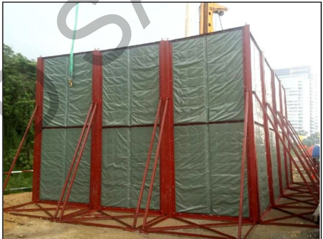
Photo 31 Example of movable noise barrier used to mitigate noise at source (Source: Guidelines for Environmental Noise Limits and Control, Third Edition, 2019 (p. 104), DOE)
