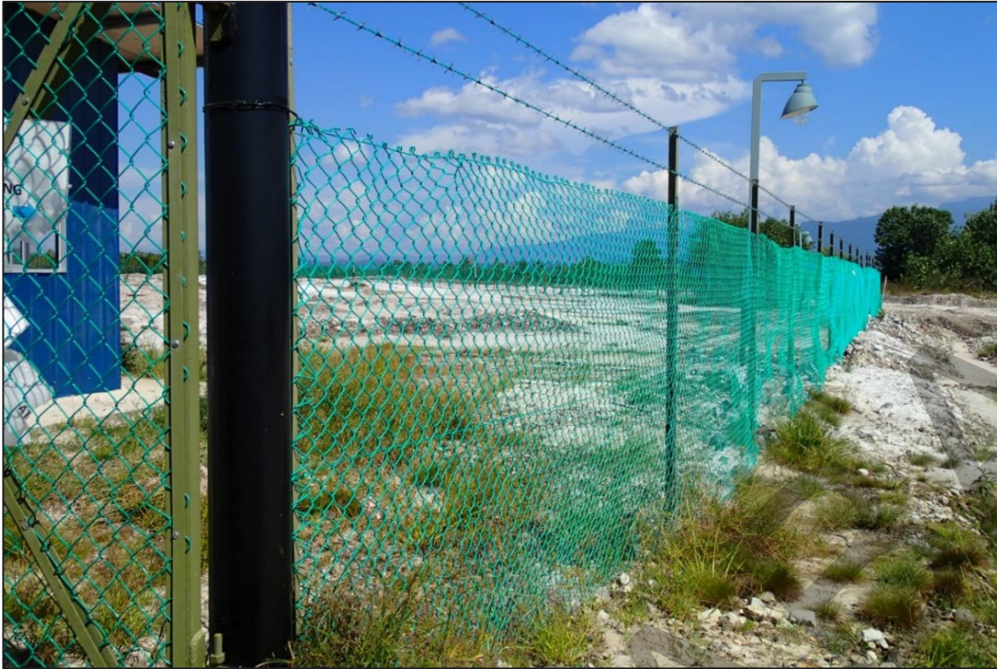
Photo 2 Example of fencing used to surround the site boundary.
