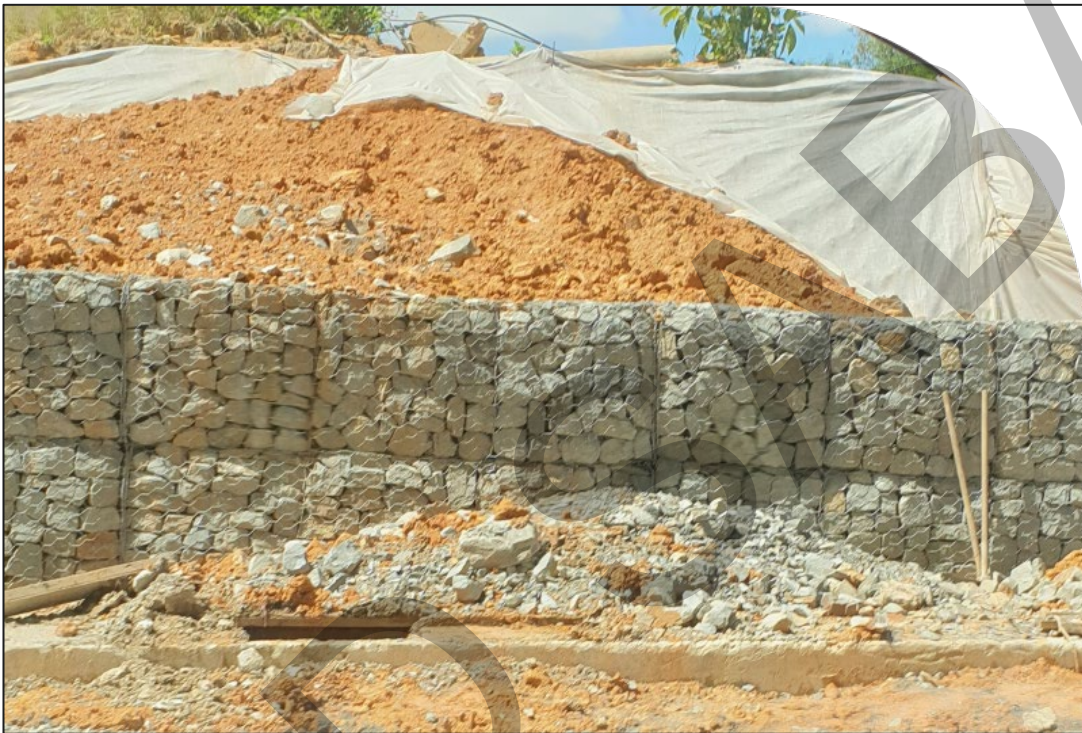
Photo 23 Soil stabilisation features using gabion structure to retain the soil.
