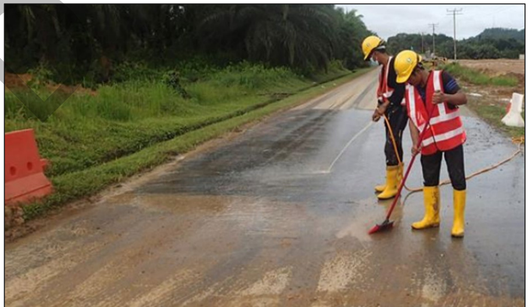
Photo 39 Example of cleaning tyres and public roads.
