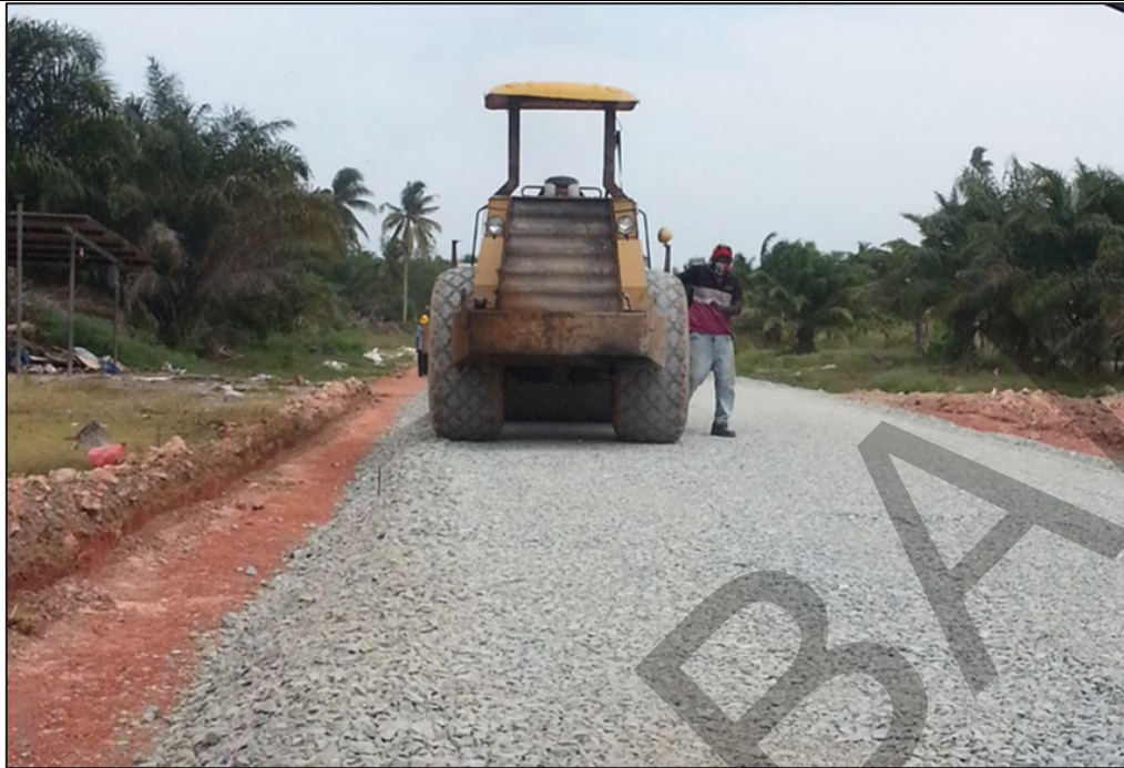
Photo 33 Example of stabilised access road using asphalt concrete.
