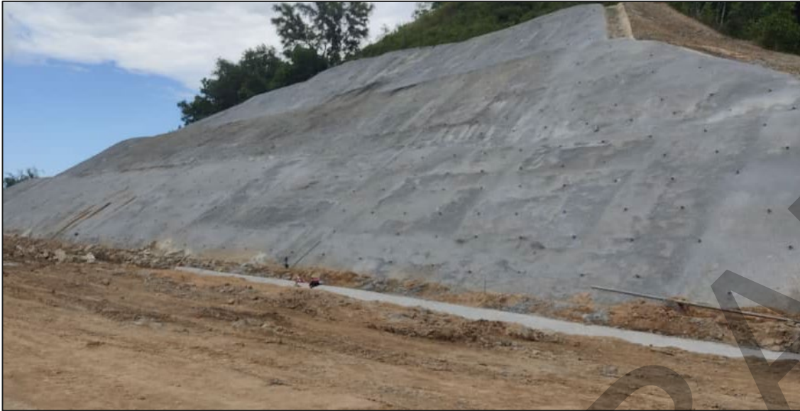
Photo 26 Example of retaining wall structure on hill slope.
