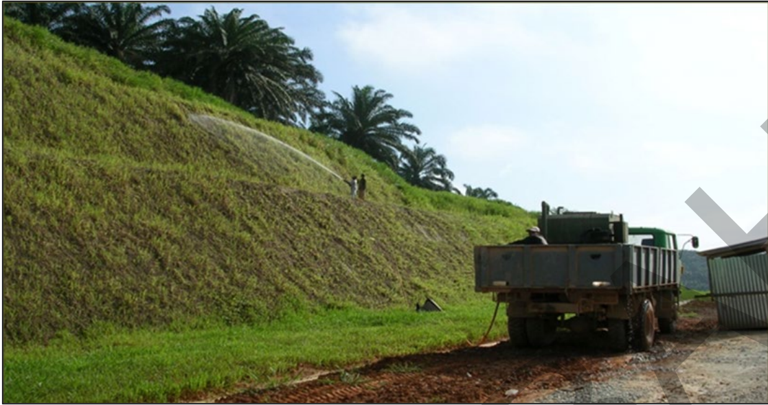
Photo 9 Example of hydro-seeding practice carried out for soil stabilisation on slope.
