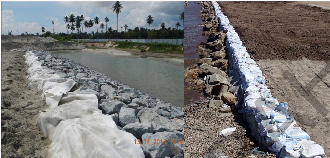
Photo 20 Example of application of perimeter bund using combination of sandbags, rocks layered with geotextile before carrying out earthwork activities.
