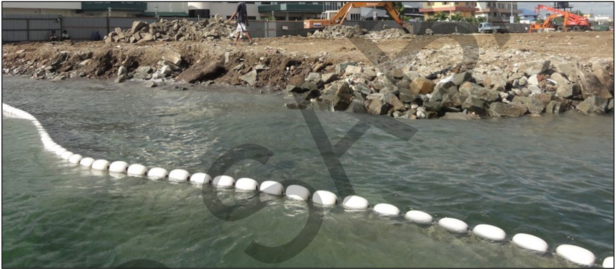
Photo 18 Example of a typical operating silt curtain.
