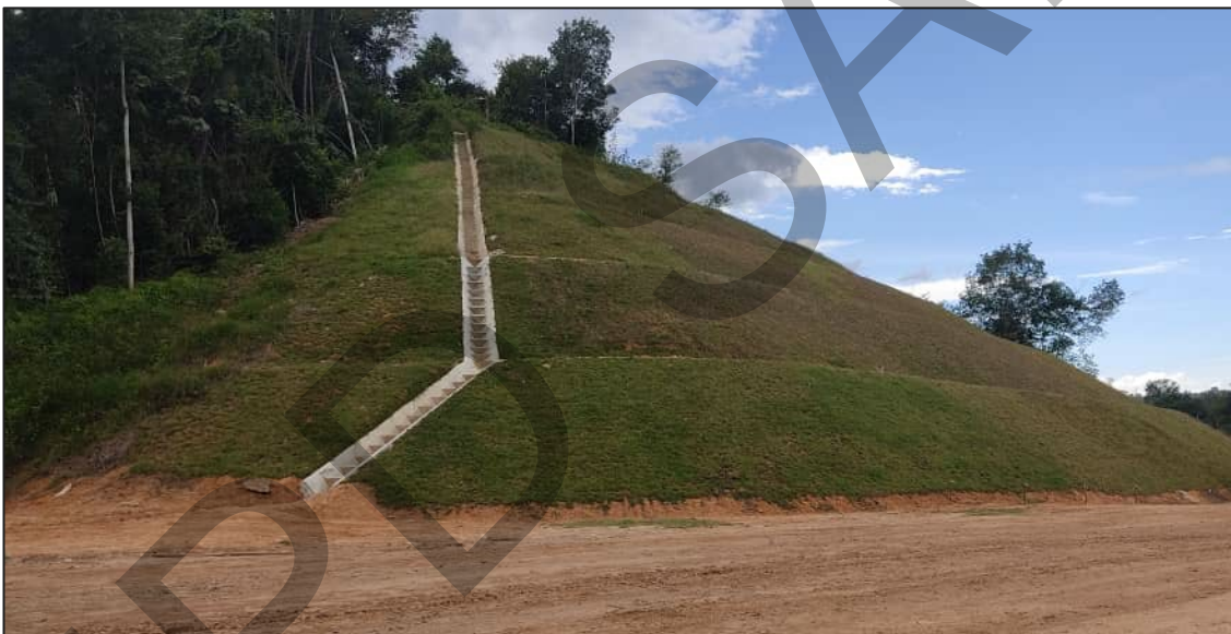
Photo 27 Example of re-vegetation such as turfing and cascading drain measures to stabilise the slope.
