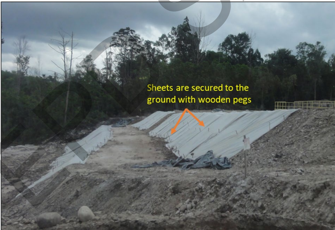
Photo 12 Example of plastic sheet covering exposed slopes and secured with wooden pegs.
