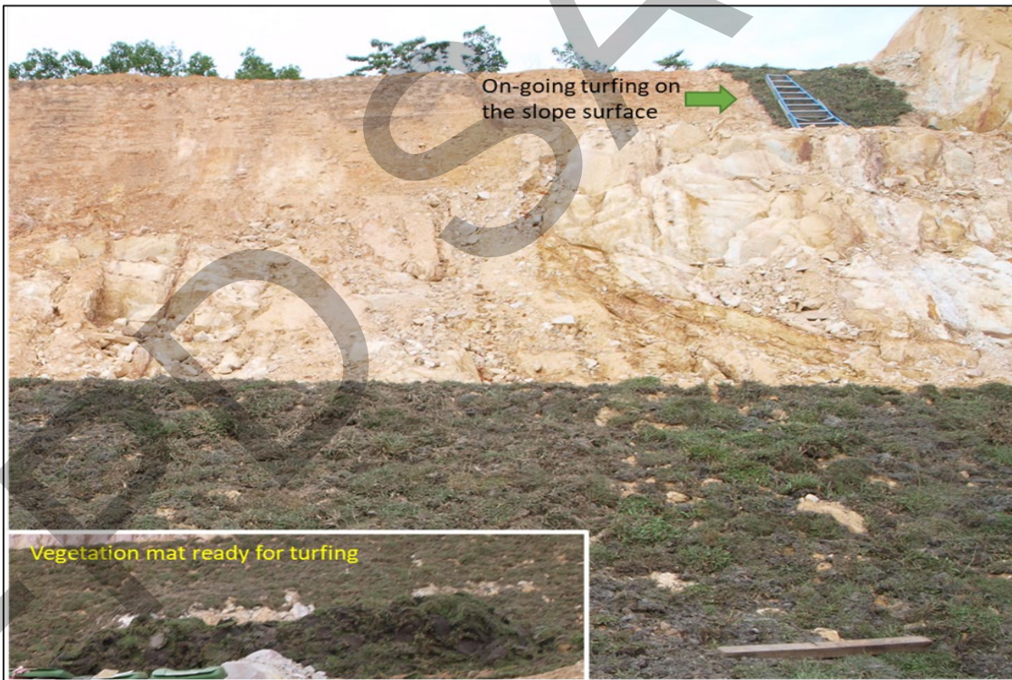
Photo 10 Turfing practice on slope surface using vegetation mat
