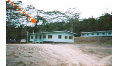
Plate 9: Existing Camp Site
