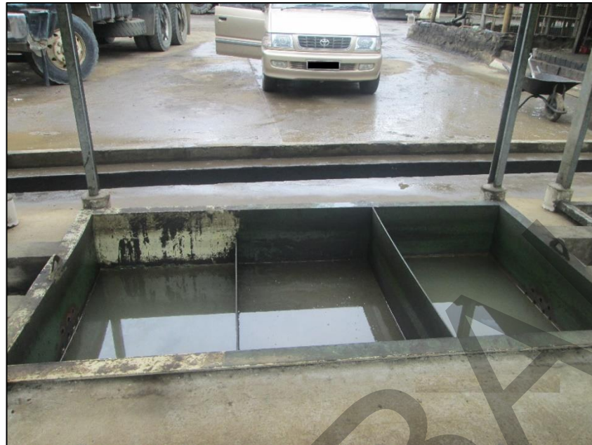
Plate 13.2: Example of oil and grease trap.
