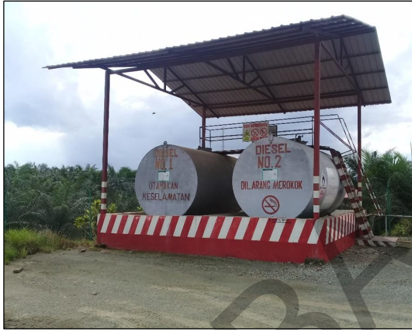
Plate 13.1: Example of permanent diesel tank with roof and bund.
