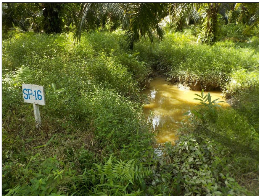
Plate 10.2: Example of silt pit constructed within the oil palm plantation.
