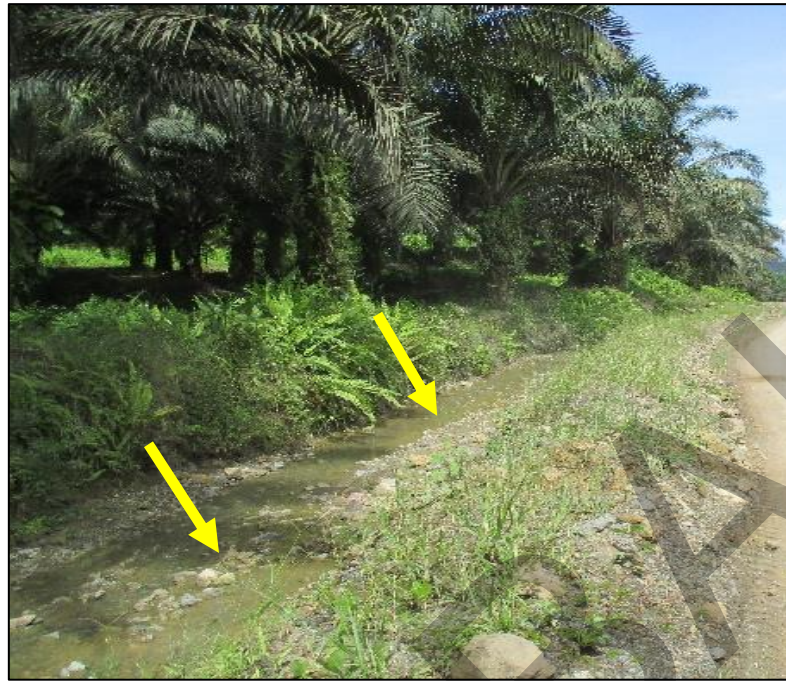
Plate 7.1: Example of earth drain provided along the road side.
