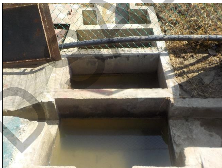
Plate 8.4: Example of oil trap for workshop.
