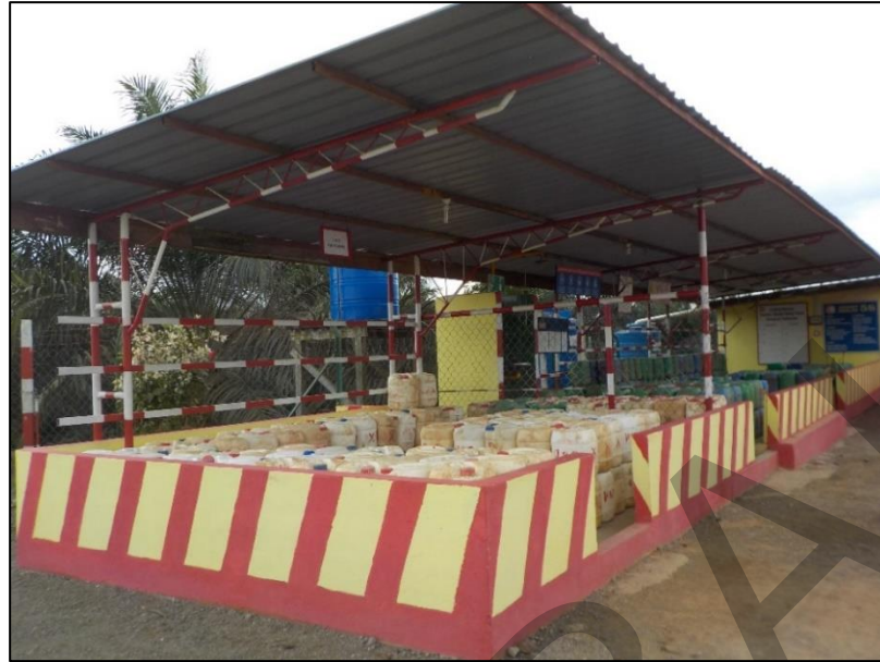
Plate 11.3: Provision of pesticides measuring and mixing area.
