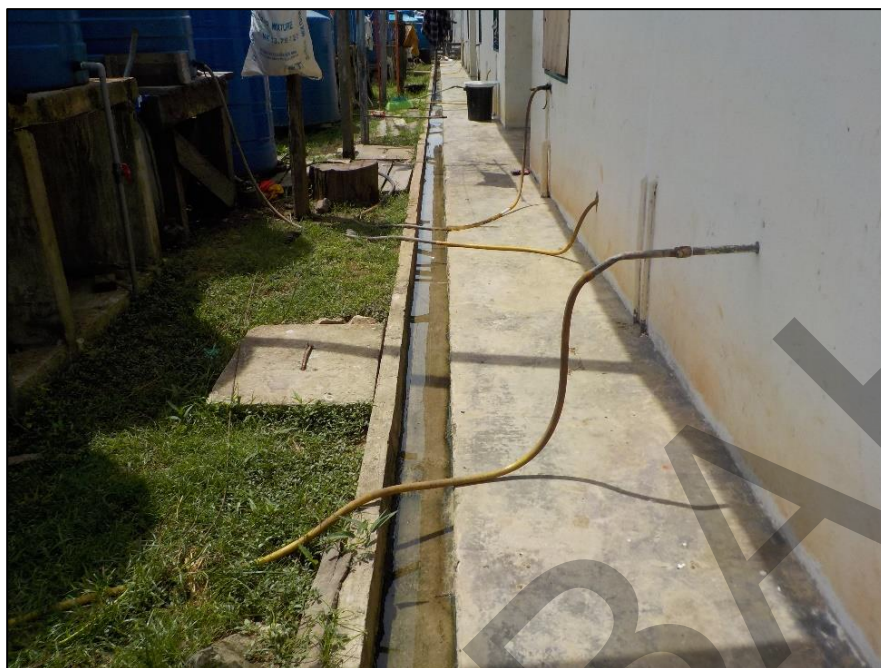
Plate 8.1: Provision of drainage system at workers quarters.
