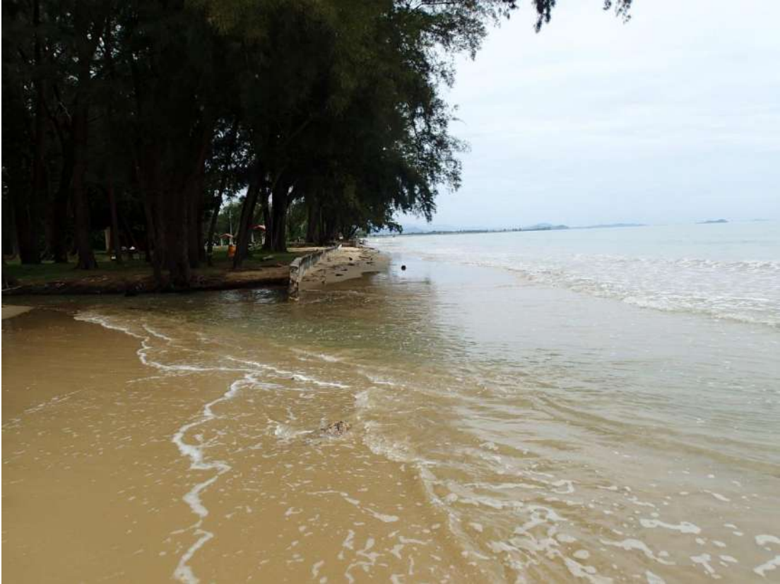
Photo 3.1 Sea encroaching behind the old seawall at high tide and covering the amenity beach
