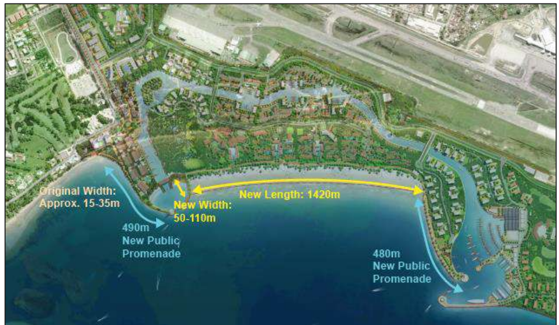
Figure 2.24 Publicly accessible waterfront areas of the Project.
