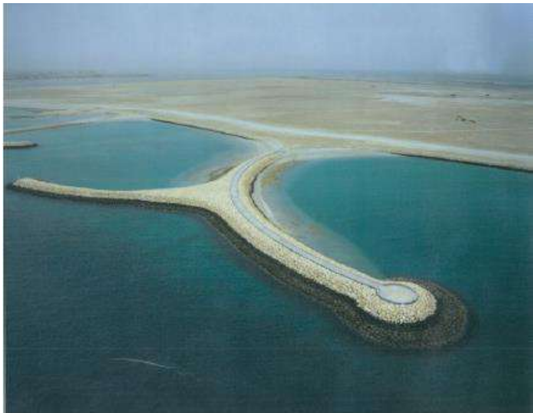
Photo 2.1 Breakwater with pedestrian access. © URS 2013.
