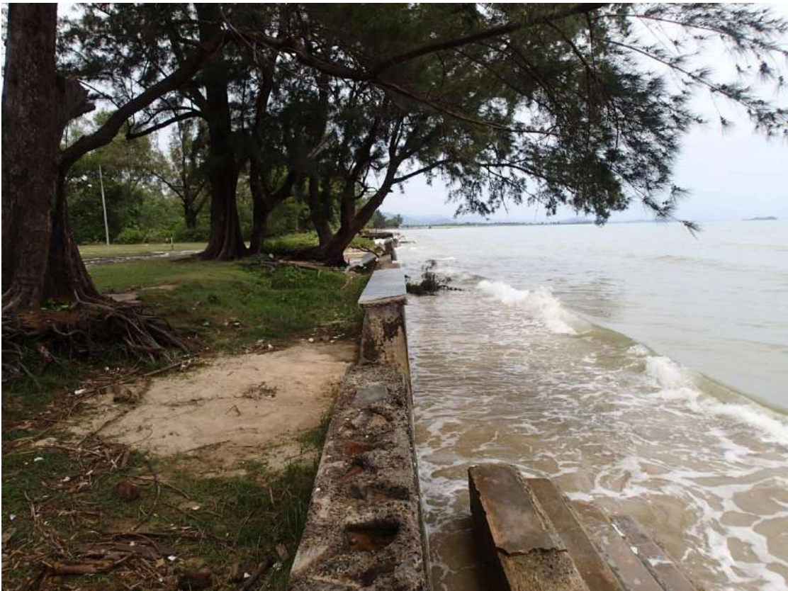
Photo 3.2 Sea encroaching right up to the old seawall at high tide and covering the amenity beach
