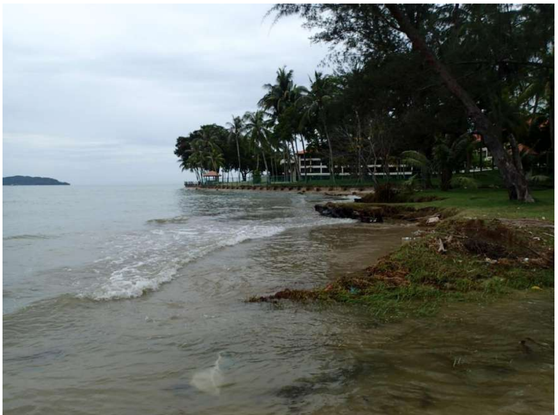
Photo 3.3 North of the project site showing the high water line reaching the grass and tree areas, there is very little margin above high water line to prevent flooding.
