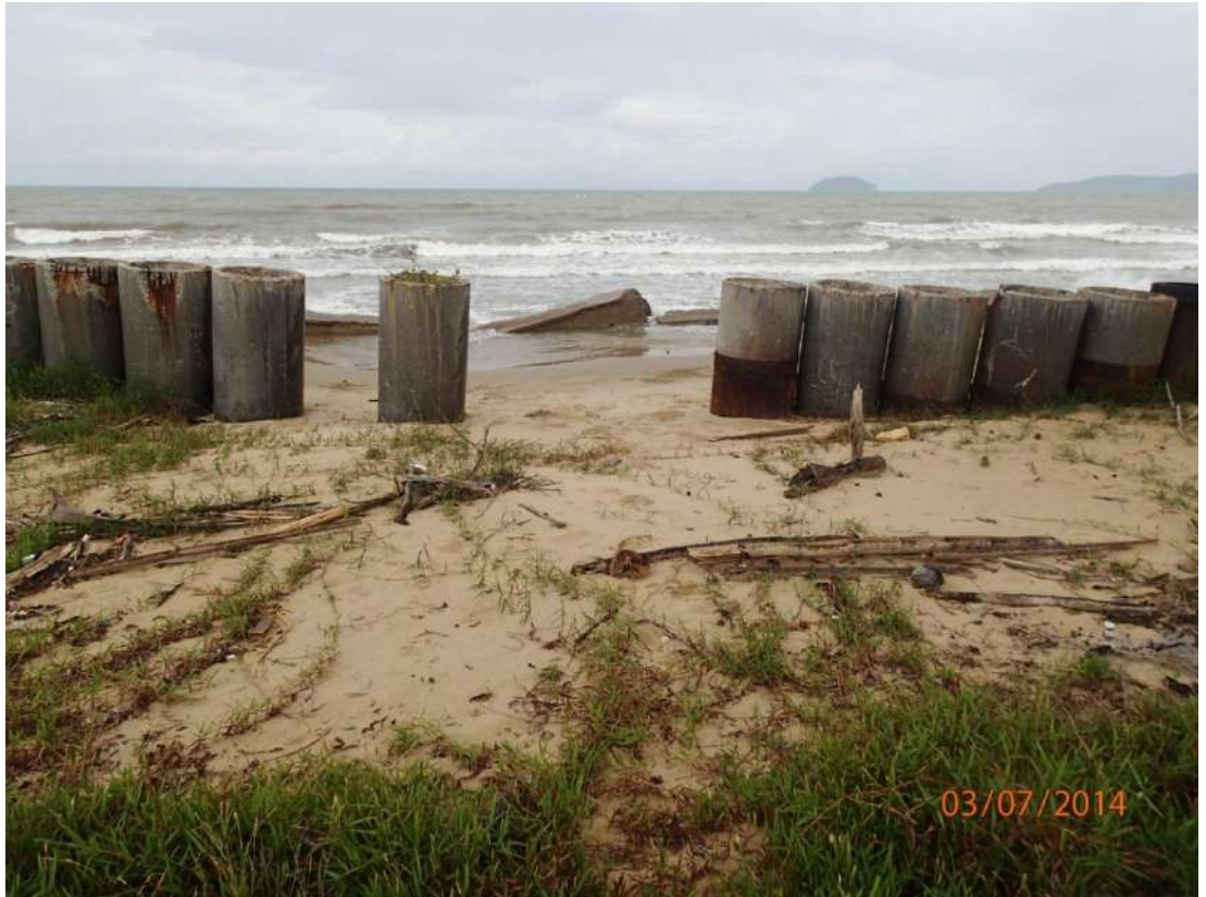
Photo 3.5 Erosion extending behind the primary line of defence and through the second line of defence (concrete piles)
