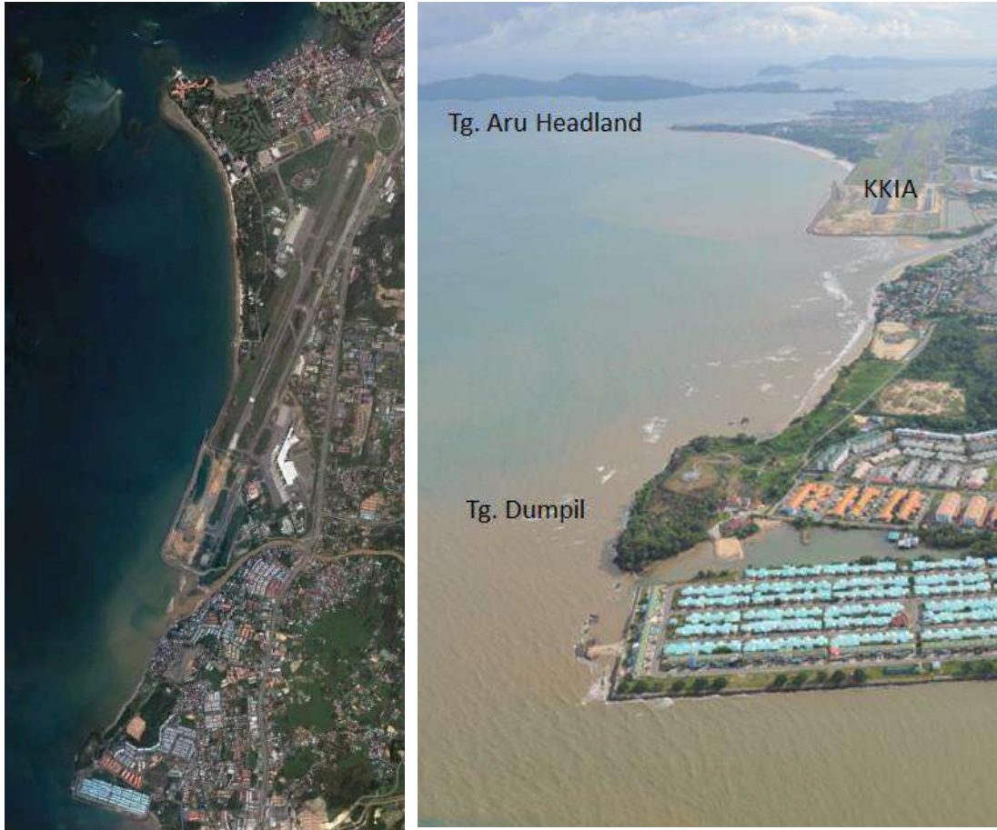
Figure 3.5 Aerial overview of Tg Aru and its features.
