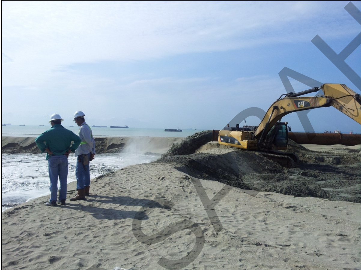
Plate 6-3: Material is pumped into phased segments or sediment basin within the reclamation area
