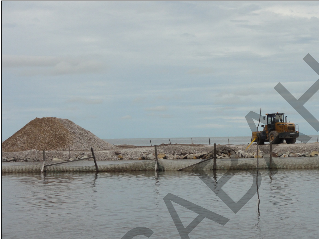
Plate 6-4: Use of silt curtains can be appropriate in low energy environment but needs regular inspection and maintenance
