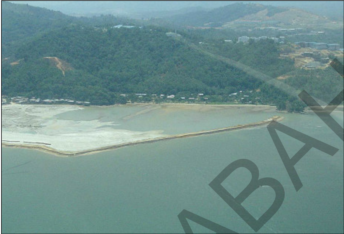
Plate 6-1: Construction of bund wall prior to filling with marine sand
