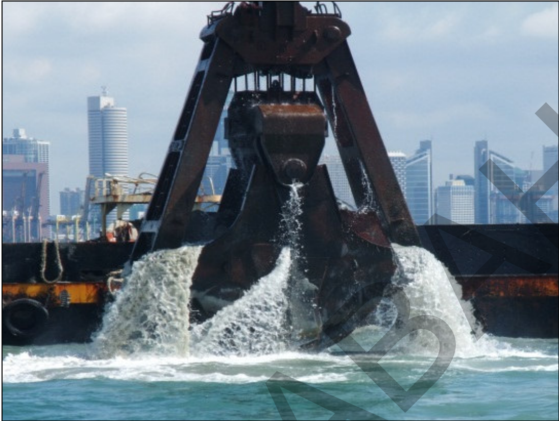
Plate 3-1: Clam shell dredger
