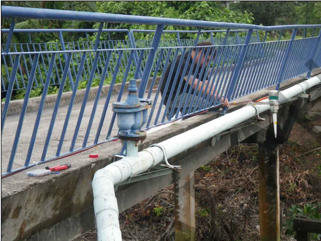
Plate 7-1: Continuous water level recorder can be established at potentially affected rivers and streams
