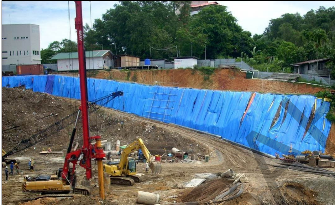
Plate 6-3: Use of canvas sheet as temporary soil erosion control onsite
