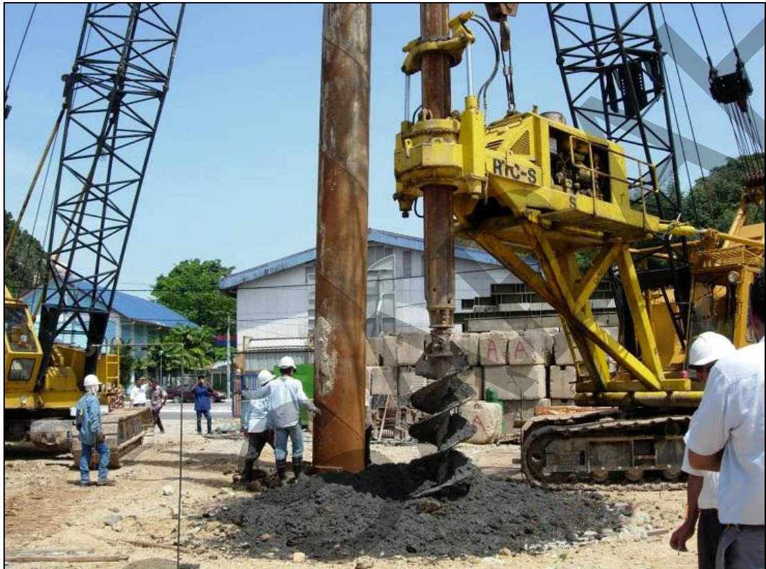
Plate 5-3: Use of bored piling for foundation works
