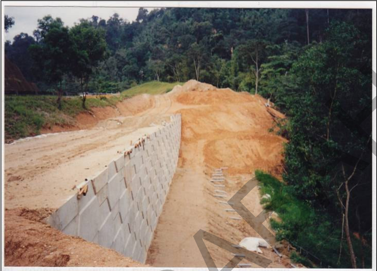
Plate 6-1: Constructed reinforced soil wall for slope strengthening
