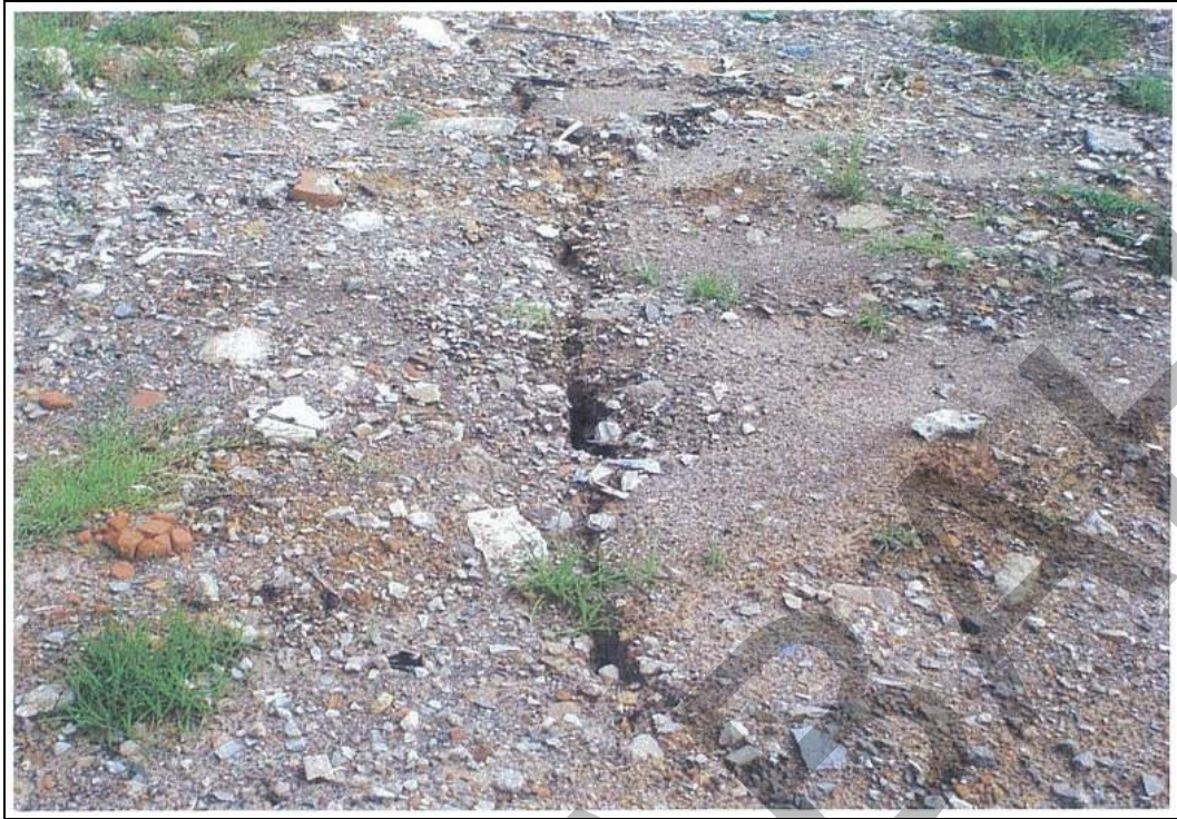
Plate 5-2: Sign of slope movement as suggested by tension cracks
