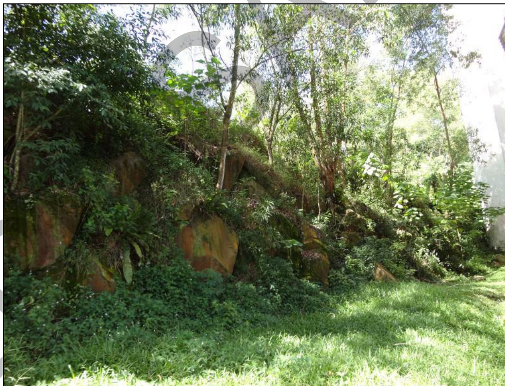
Plate 5-1: Tilting of trees and failing boulders are common signs of slope movement
