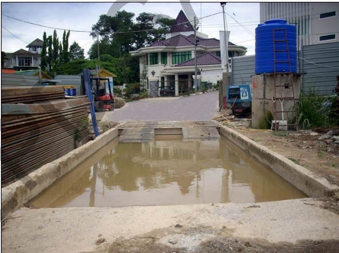
Plate 6-4: Wheel washing bay with water spraying facilities within a construction site
