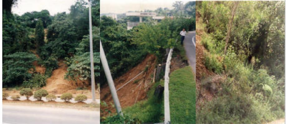
*Photo 2.5 Debris avalanche from a landslide on steep slope. Photo 2.11 Landslide affecting road built on slope Photo 2.7 Active slide as suggested by the slanting of trees*
