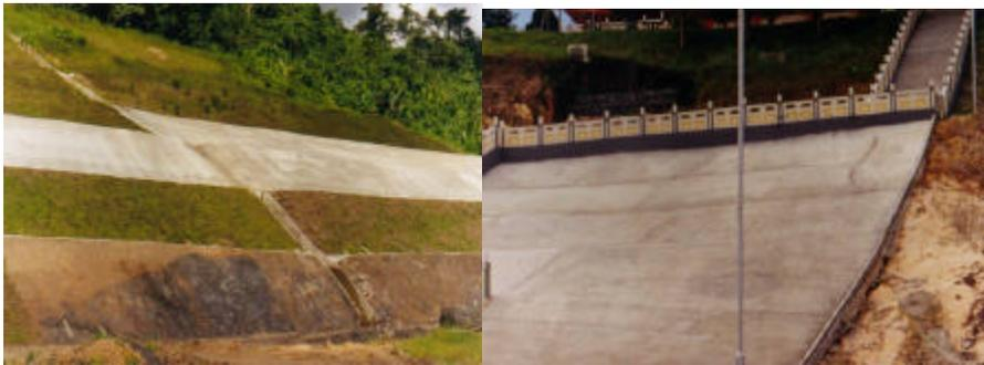
*Photo 3.5 Combination of gunite and turfing Photo 3.6 Cement mortar rendered slope protection*
