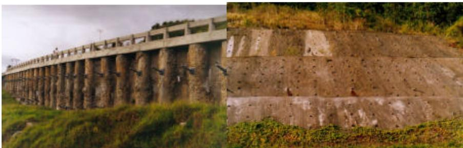
*Photo 3.7 Anchored bored-pile wall Photo 3.8 Slope protected by gunite wall*
