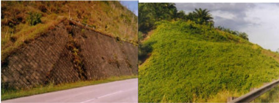
*Photo 3.3 Reinforced Concrete wall protecting cut slope Photo 3.4 Soil slope protected by creepers*
