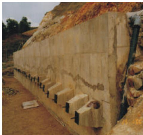
*Photo 3.2 Rock slope protection using anchored tie wall*
