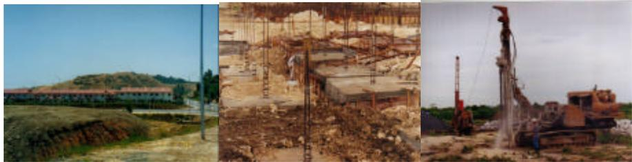
Photo 1.1 Clearing of project site Photo 1.2 Laying of pad footing Photo 1.3 Micropiling
