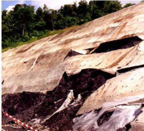
*Photo 3.9 Slope failure*
